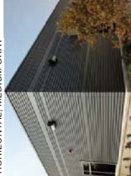
MP-2 CONCEALED-FASTENER METAL WALL PANEL SYSTEM, HORIZONTAL, MEDIUM GRAY
