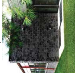
CML-2 FULLY GROUTED CONCRETE MASONRY BLOCK, ROUGH FINISH, DARK COLOR
