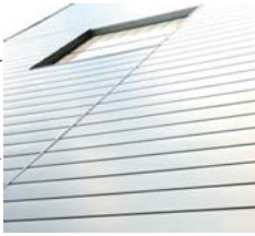
MP-1 CONCEALED-FASTENER METAL WALL PANEL SYSTEM, VERTICAL, OFF-WHITE (BONE WHITE)
