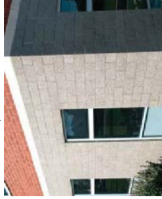
CML-1 FULLY GROUTED CONCRETE MASONRY BLOCK, SMOOTH FINISH, LIGHT COLOR
