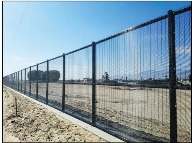
Figure 1: Welded wire anti-climb metal fence
