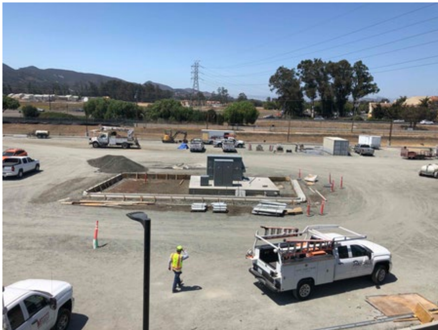
View of the utility yard and transformers for Phase 1 of the Battery-Electric Bus recharging system. At the western edge of the bus parking area, you can barely see the conduits sticking up from the ground for future Phase 2 improvements.
