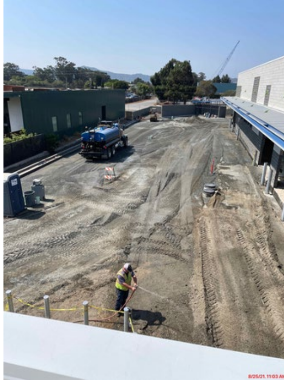
Rough grading of the bus entrance drive aisle between the back side of the maintenance bays and the main CAPSLO building on the left (looking southbound from the roof over the parts unloading area). The SLO City Corp Yard can be seen in the distance.
