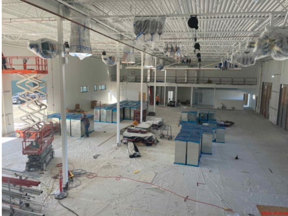
View of bus maintenance bays from the northern storage mezzanine, with the southern storage mezzanine at the far end. Much of the overhead equipment is still wrapped in plastic during this painting phase, and the air-handling ducts stacked on the floor await installation.
