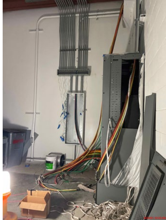
Pulling wire from the electrical room on the northern storage mezzanine to the other side of the Shop feeding the maintenance bays. The REALLY big cables run to the bus recharging area (see below) from the main electrical room located in the Administration area.
