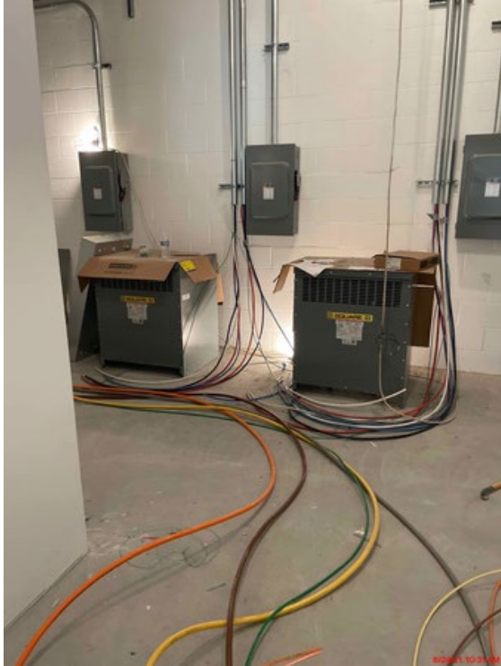
Pulling wire from the electrical room on the northern storage mezzanine to the other side of the Shop feeding the maintenance bays. The REALLY big cables run to the bus recharging area (see below) from the main electrical room located in the Administration area.
