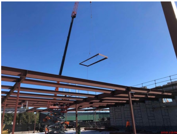
Crane loading structural steel
