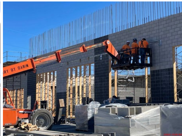
Installation of CMU embeds on exterior of shop doors
