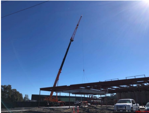
Crane installing public entrance structure
