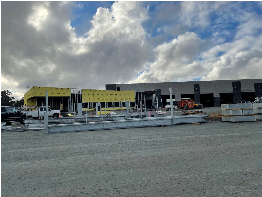
Installation of shear wall and insulation sheathing on the Dispatch portion of the operations/administration building on April 26 th , looking due East from the bus parking area
