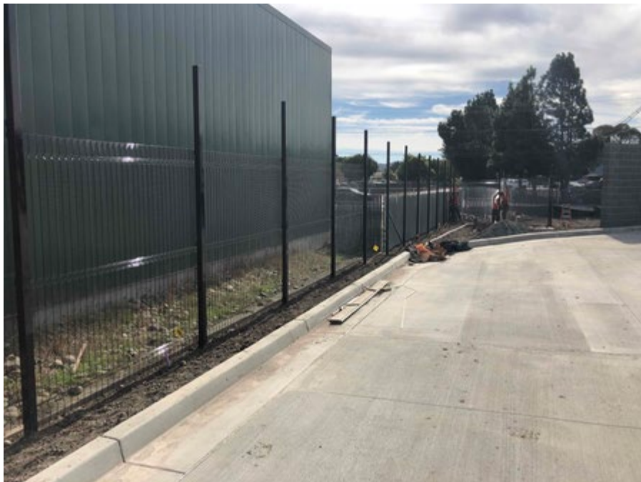
Anti-climb fencing being installed (prior to trimming of the vertical posts). This fencing will surround the entire project site.
