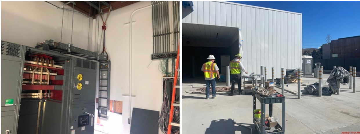
View of the infamous Electrical Bus Duct system, snaking its way from the building penetration and terminating at the top of the main electrical panel. The picture to the right shows where it penetrates the building; PG&E will place the main transformer on the adjacent concrete pad that is surrounded by the steel bollards and connect the transformer to the Duct during the week of November 29 th .
