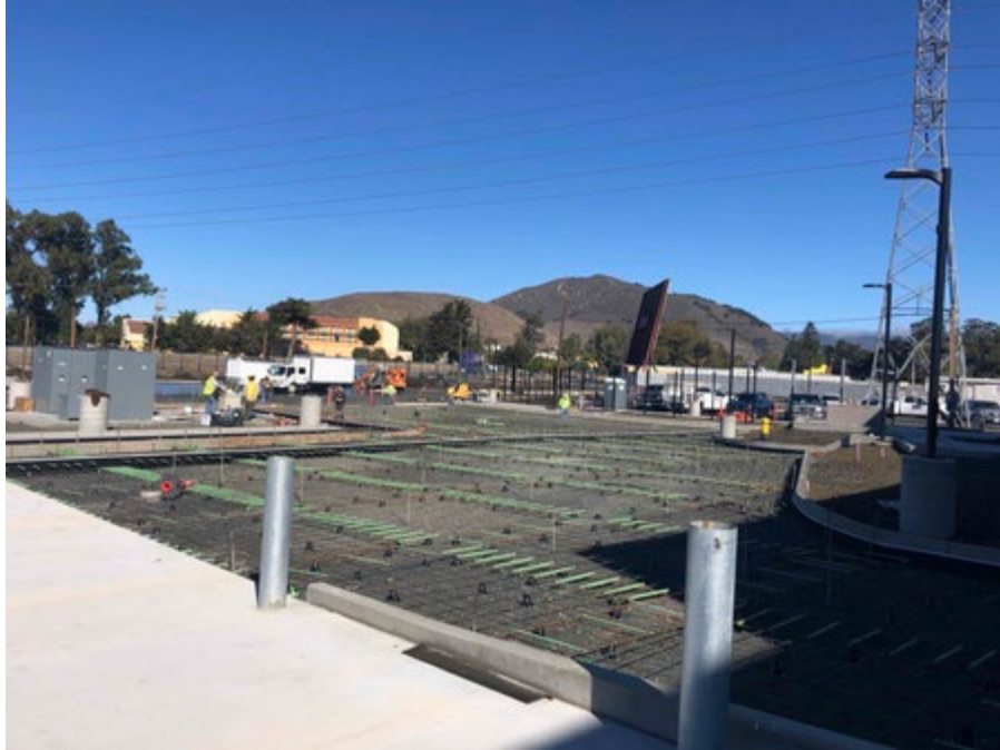
October 25 th view of rebar being placed prior to a ~200 cubic yard concrete pour planned for October 27 th . Pours will be completed every few days to complete this important phase of the work.
