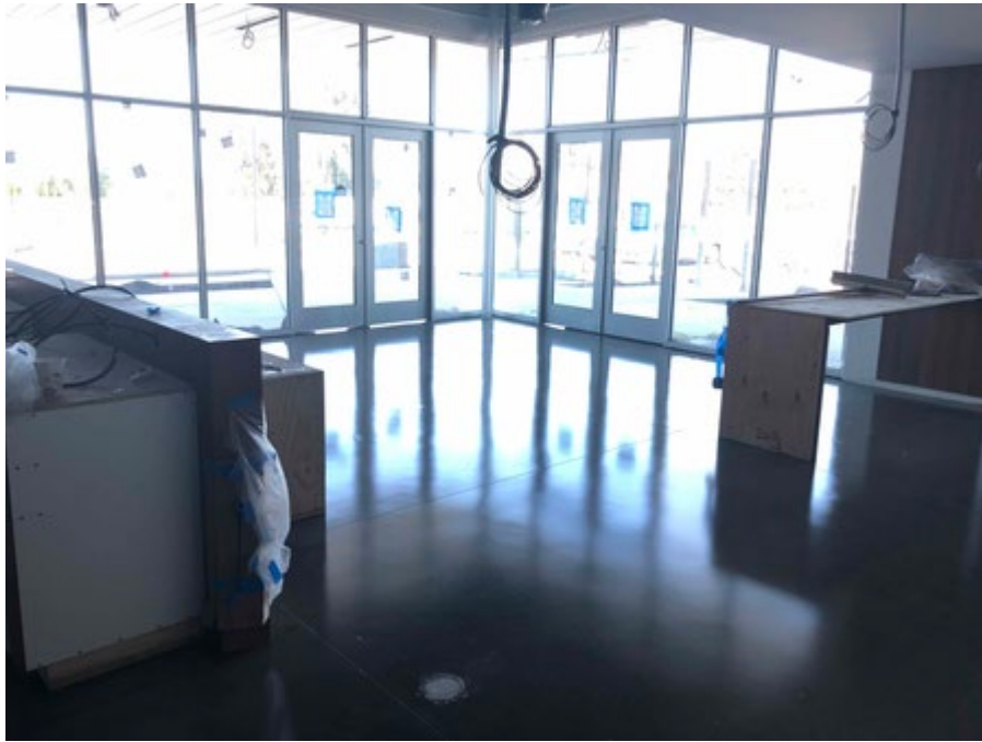
View of polished concrete in the employee break room. Crews came in over the weekend to complete this work in order to allow other trades (electrical, communications, HVAC, etc.) to work unhindered during the workweek.
